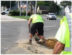
Backfilling required the use of a "Jumping Jack" compactor. The worker was properly attired in the high visibility safety vest, Safety Glasses, hearing protection, and Work gloves with leather palms & fingers cloth uppers. The operator was cautious to keep his feet from the moving compactor and was familiar with the operation of the tool.
