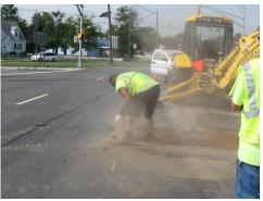
A cutoff saw was used to square the opening in the asphalt. This operation was completed without the use of water or any wetting method. Dry cutting of certain materials exposes workers to silica. This saw was equipped to be used with a water supply. According to workers, the water supply was not available for this job. The level of dust generated exceeded recommended PELs. (Permissible Exposure Limits)
